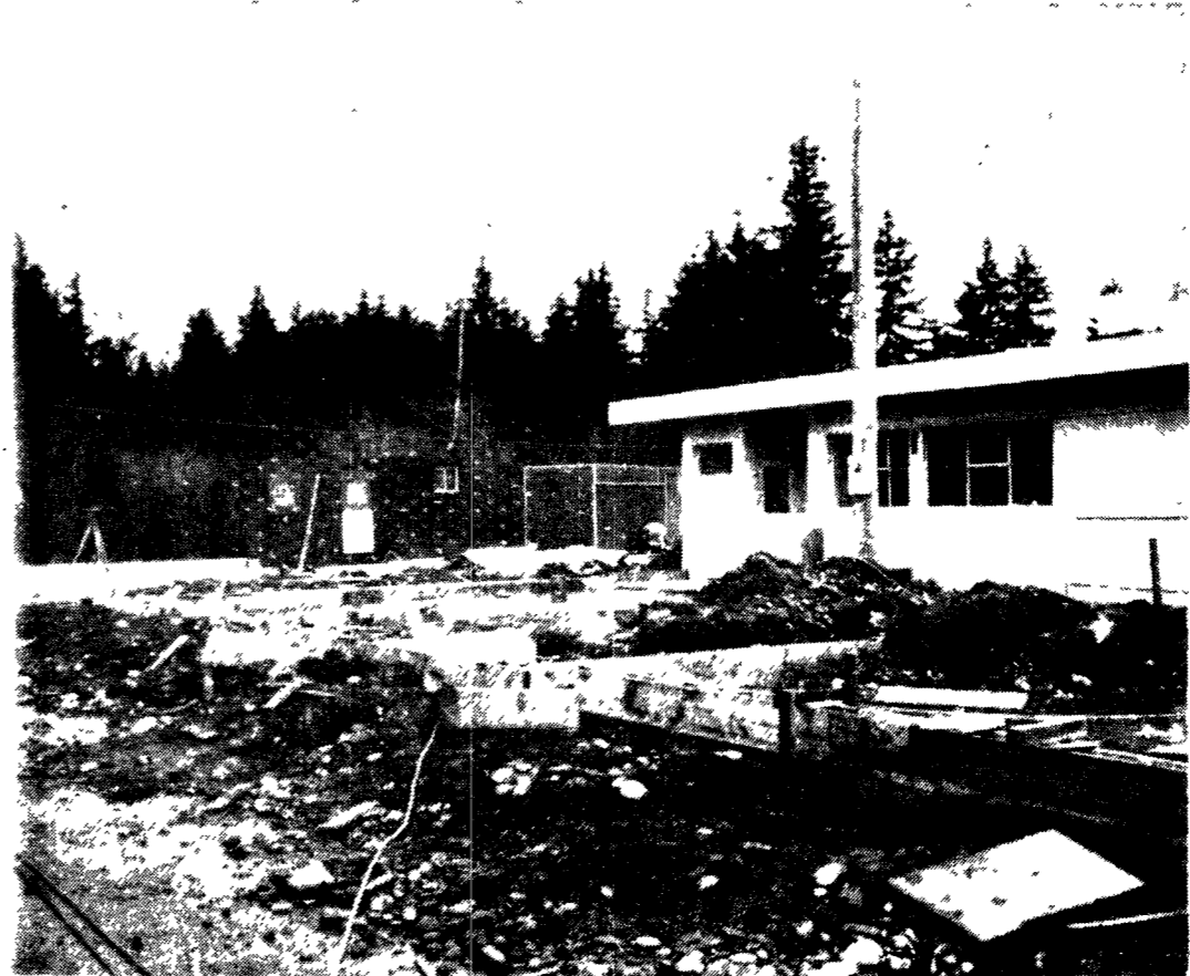
Construction is underway for the addition to the Forks Community Hospital. Wick Construction Company of Seattle received the contract from the hospital district.
